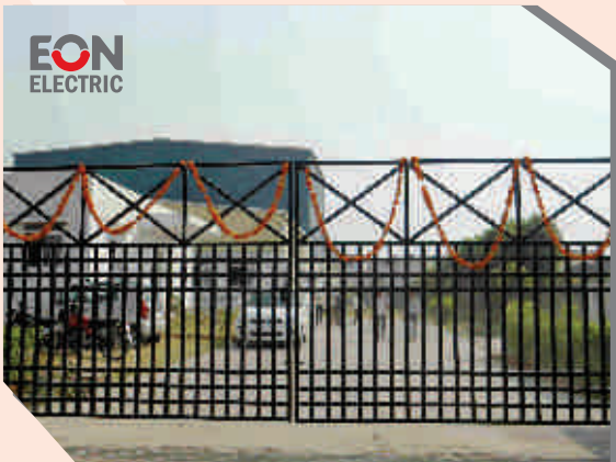
Fan Plant at Haridwar
