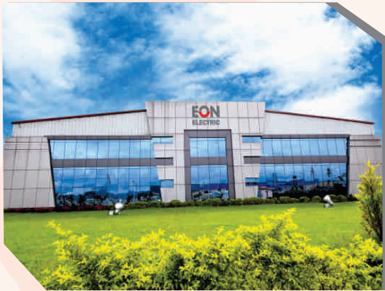
Wires & Cables & Mobile Accessories Plant at Haridwar
