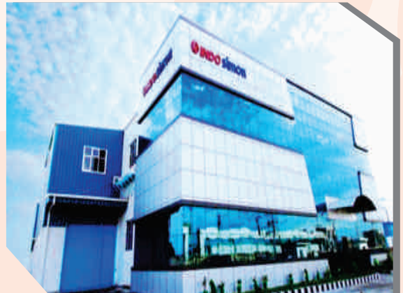
Modular Switches Plant at Haridwar
