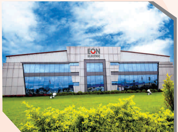
Wires & Cables, LED Lights & Mobile Accessories Plant at Haridwar
