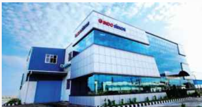
Modular Switches Plant Haridwar
