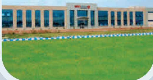
Switchgear Plant, Haridwar
